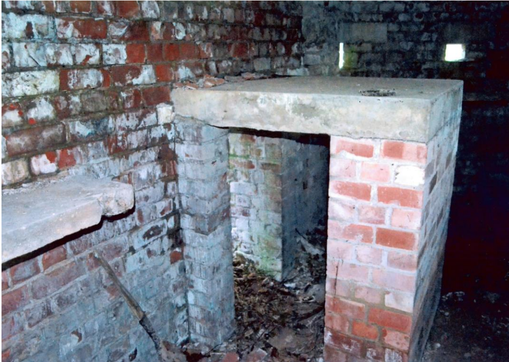
Fig 2: Internal Blast wall, Sturrock's Farm Pillbox (photo D Self)
