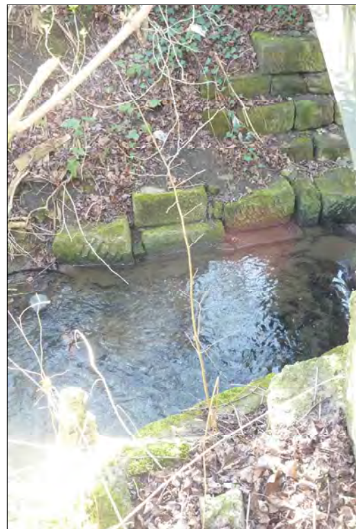
Stone revetment of leat by Rainton footbridge
