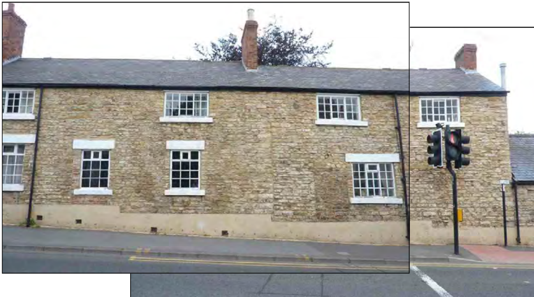
Blocked doorways, windows, butt joints etc
