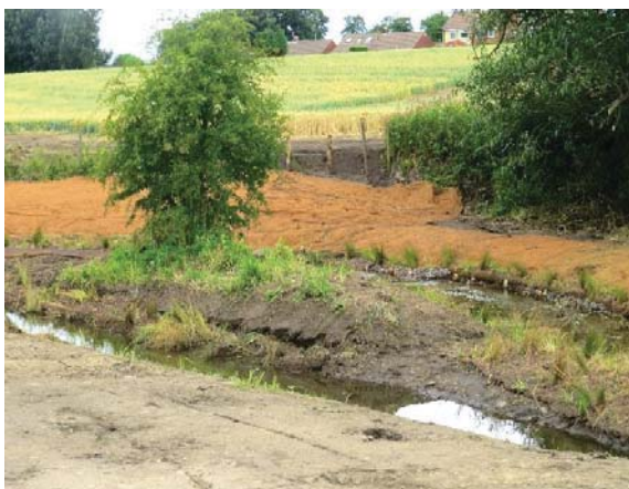
Stream re-alignment and restoration of banks
