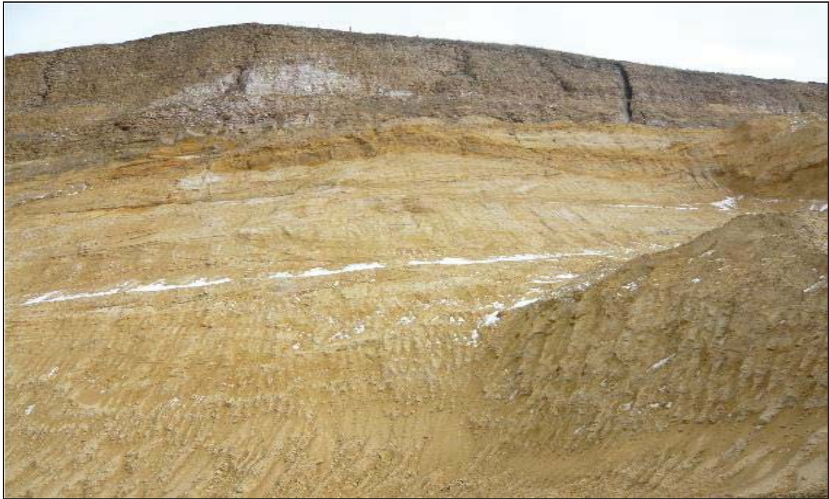
This photograph taken in April 2013 shows the working Eppleton quarry. A large yellow sand dune can be seen and above it the Magnesian Limestone rock (Dolomite) with vertical fissures (cracks) extending down the face. The vertical striations in the sand are caused by machinery working during extraction. This winter picture also shows snow.
