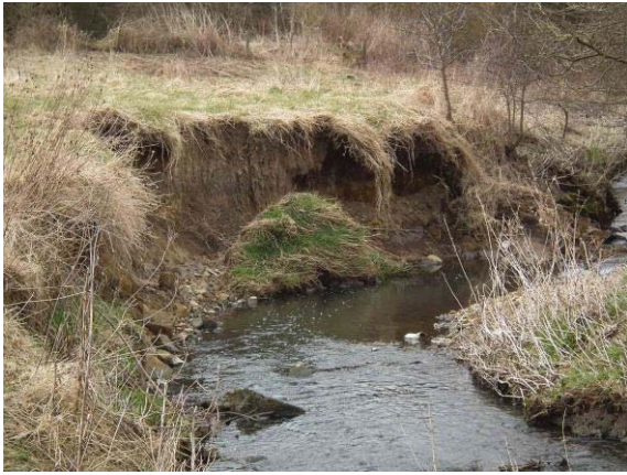
Recent heavy rainfall has increased the likelihood of bank erosion
