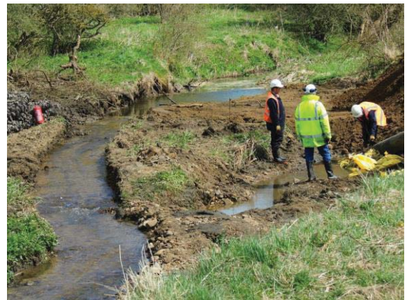
Reclamation and stream re-alignment follows the flooding
