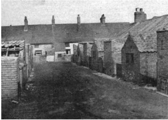
The single storey cottages in the Brickgarth at Easington Lane were replaced with 2 storey houses. Note the windows neatly tucked beneath the eaves. Each house had a back yard, giving some privacy in which could be found an outside toilet and a coalhouse and sometimes a wash-house. Most of these houses were demolished during the 1950s.
