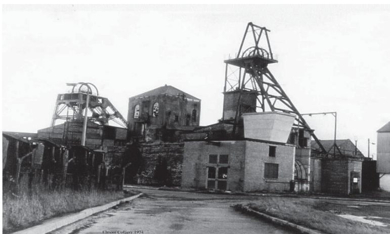
Elemore colliery in 1974 showing the small funnel of the early fan together with the fan house. Note the double winding wheel on the George headstock to the left.
