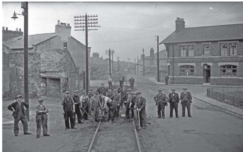
Lifting the track in Railway Street Hetton in 1959
