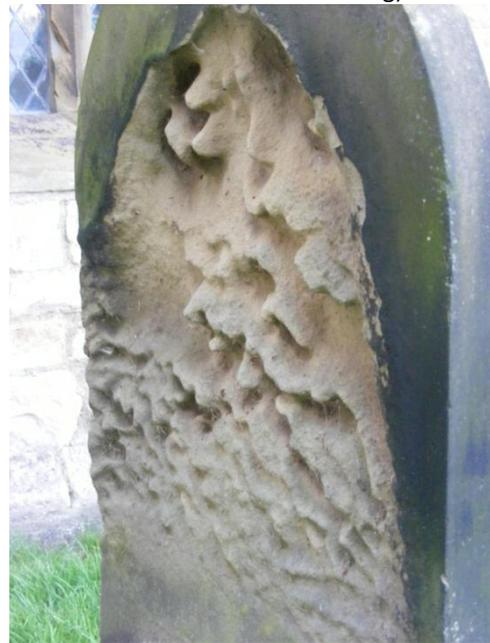
Sandstone grave marker showing effects of 'acid' rain
