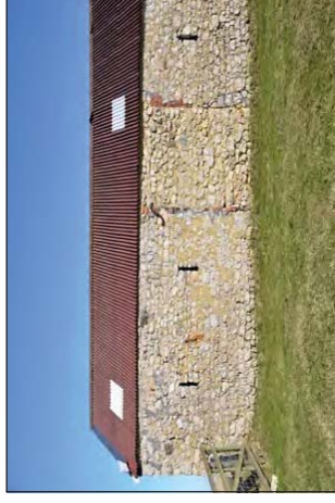
Building analysis - note blocked opening in the wall.
