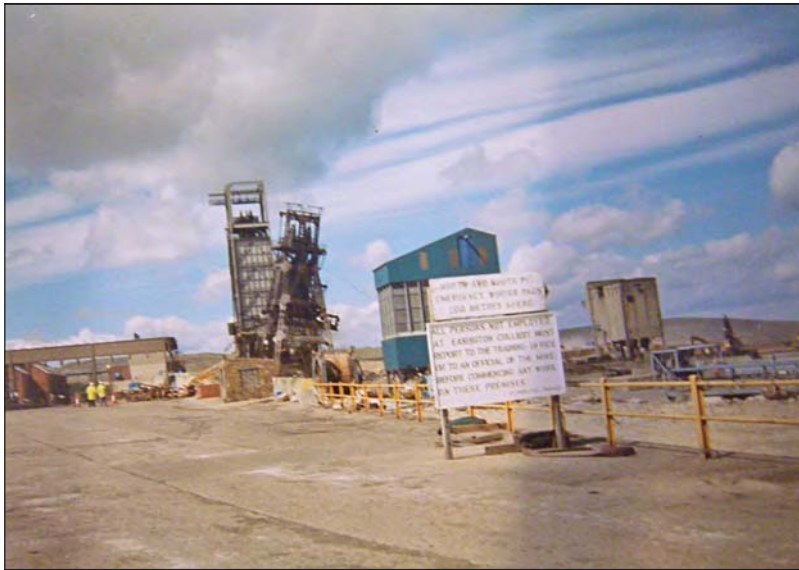
Demolition of the winding gear after closure
