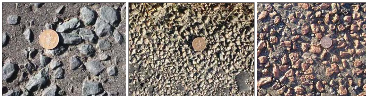
Plates 58 to 60: Crushed rock used in Cleadon's road surfaces – (left to right) Whin Sill dolerite chippings in the surface of Whitburn Road, Shap Granite chippings in Cleadon Hill Lane and distinctive red microgranite from Harden Quarry in north Northumberland, which gives a distinctive colour to Marsden Road.
