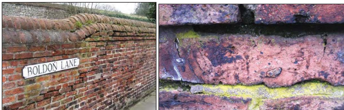
Plates 43 and 44: The beautifully constructed brick wall at Cleadon House features a finely shaped brick coping, and detail of boundary wall, showing sandstone clasts in brick.
