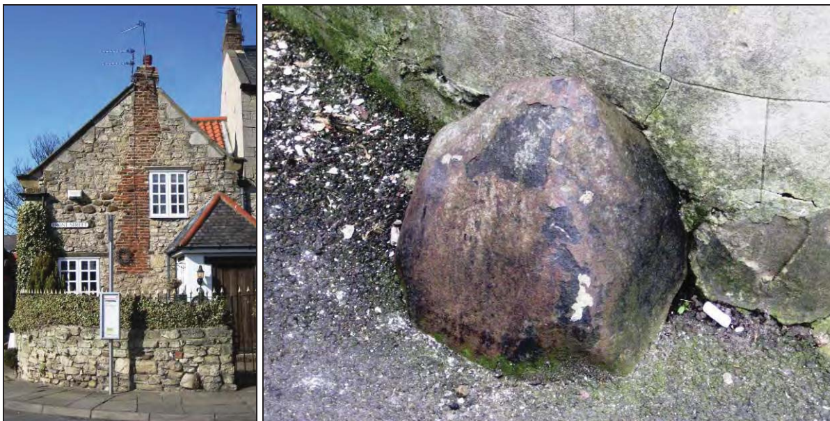
Plates 33 and 34: Front Street - The old Methodist chapel cottage incorporates a variety of building materials. The bulk of the walls are formed of local limestone rubble, though dark brown erratic boulders of Whin Sill dolerite are conspicuous, especially above the street name plate. Coal Measures sandstone blocks are used in the skewes and cappings of the gable wall. Brick, almost certainly made from locally dug clay, marks the external course of the flue; and an erratic boulder of Whin Sill dolerite used as a cart stop in the foundation of a shop on Front Street.
