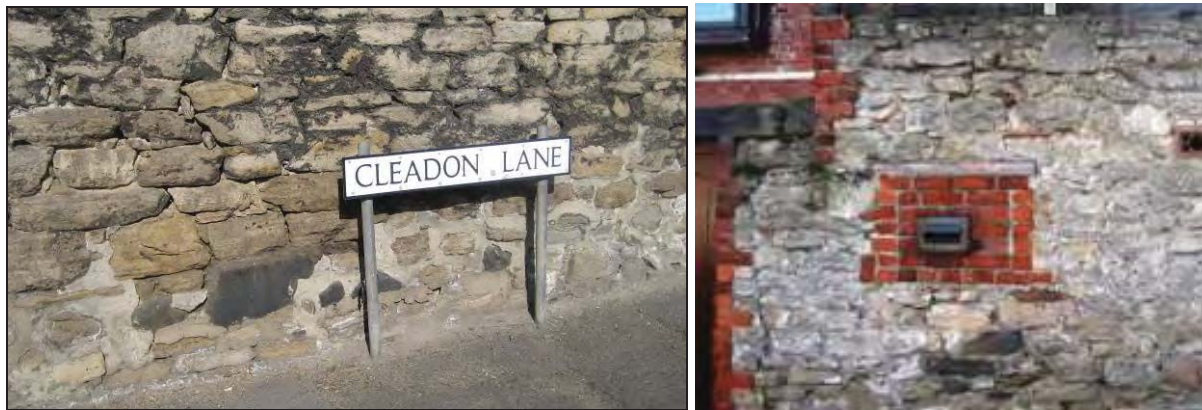
Plates 53 and 54: Boundary wall in Cleadon Lane built of local limestone with conspicuous glacial erratic boulders of dark grey Whin Sill dolerite, and wall in North Street, built predominantly of local limestone, but with erratic blocks of dark brown Coal Measures sandstone and dark grey Whin Sill dolerite conspicuous below the letter box, as well as re-used brick.
