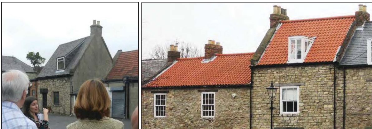
Plates 47 and 48: Steep pitch of the florist's shop on Front Street would suggest that this building was once thatched, and the modern pantiled roofs contrasting with the Welsh slate of the building north of the pond, formerly part of Burdon farm.
