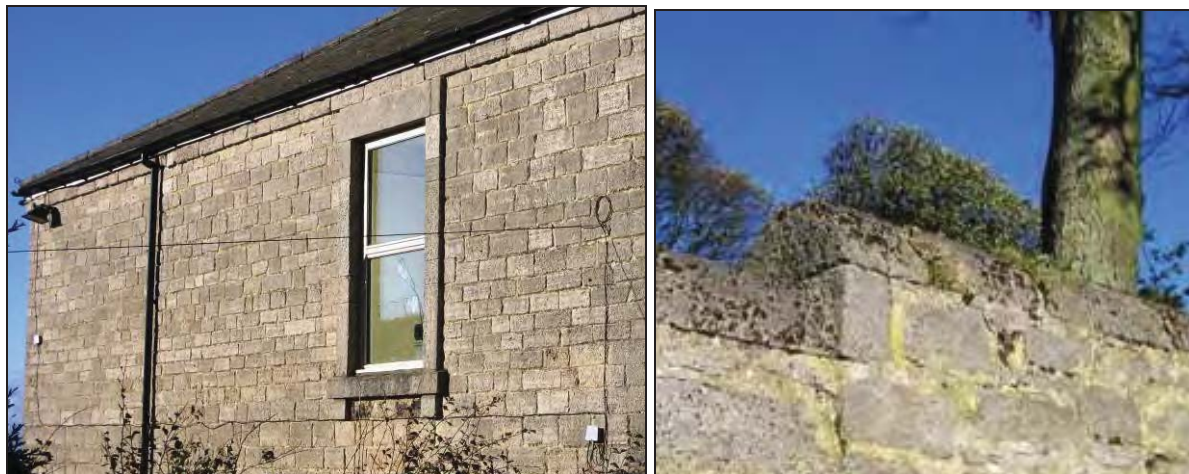
Plates 31 to 32: Sunnyside Farm - a rare example of construction using squared blocks of local limestone and the same material used nearby in the coping stones of the Waterworks boundary wall
