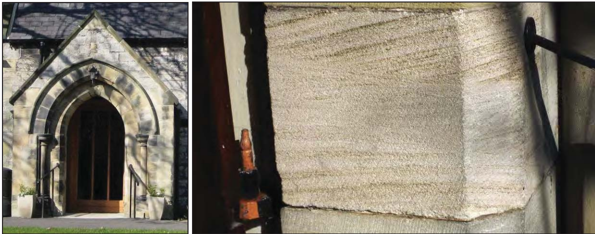
Plates 38 and 39: All Saints Church - Coal Measures sandstone used in the door mouldings, and detail of coarse-grained Coal Measures sandstone showing that this block is inverted.
