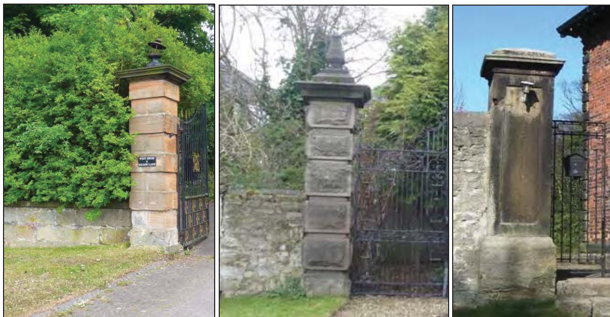
Plates 55 to 57: (Left to right) Cleadon House, gates south of the pond and Cleadon Waterworks - three of Cleadon's fine gateposts, all built of imported sandstone, the source of which remains unknown but is likely to be from quarries in northern England. The colour and nature of the stone in each is slightly different.
