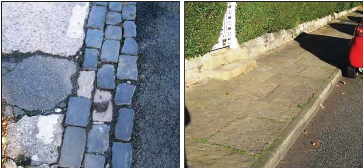
Plates 61 and 62: Whin Sill dolerite (dark grey) and granite (pale grey) setts in North Street, and the pavement in Front Street, which is built from sandstone slabs of unknown provenance.
