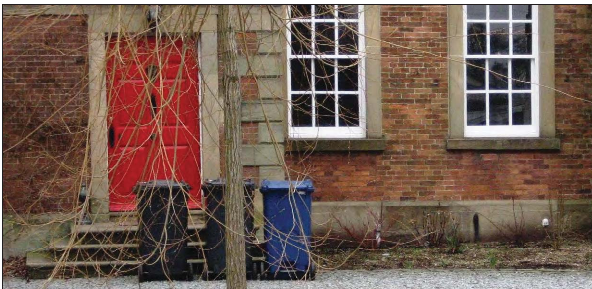
Plate 42: Cleadon House – built of locally produced red brick with Coal Measures sandstone used for window and door casings.
