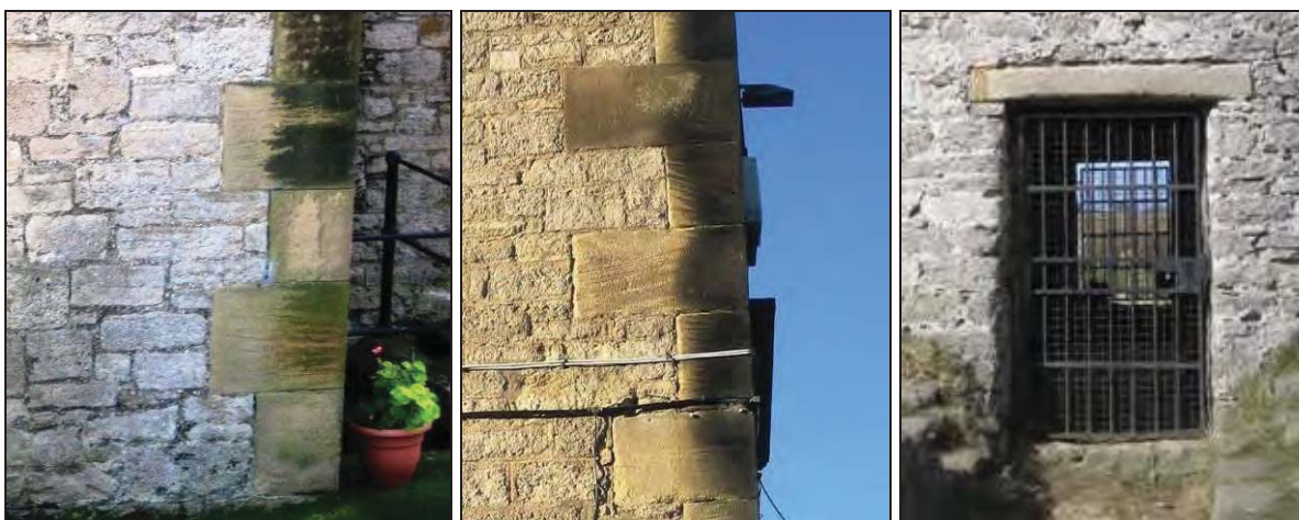
Plates 35 to 37: (left to right) All Saints Church - the quoins are of sandstone, almost certainly from the Coal Measures. Cross-bedding, accentuated by weathering, is conspicuous in the block second from the ground. The Britannia Inn - sandstone, almost certainly from the Coal Measures, forms the quoins. Cleadon Windmill - the door lintel is a large slab of pale buff, cross-bedded sandstone, almost certainly from the Coal Measures
