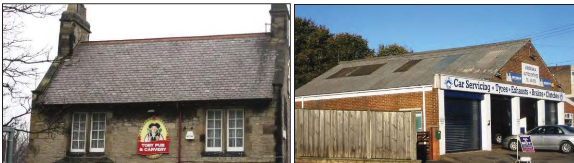
Plates 49 and 50: Welsh slate roof of the Britannia Inn, and Britannia Autoservices, roofed with sheets of corrugated asbestos cement.
