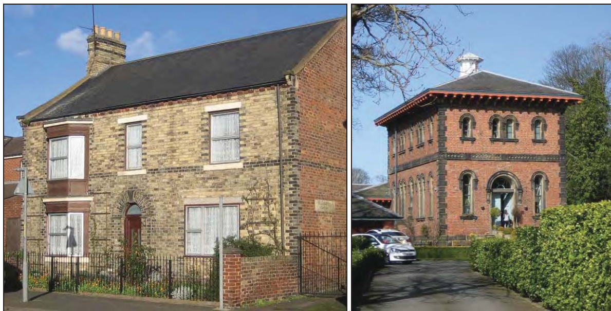
Plates 45 and 46: Grove House, the front elevation of which is built of pale cream firebrick made from Coal Measures fireclay. Cleadon Waterworks, made of machine made brick with Sandstone detailing in the window and door casings, quoins and as the string course.
