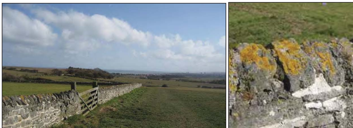
Plates 51 and 52: Field boundary wall on Cleadon Hills, and detail of the worked stone capping, a rare example of shaping the local limestone.
