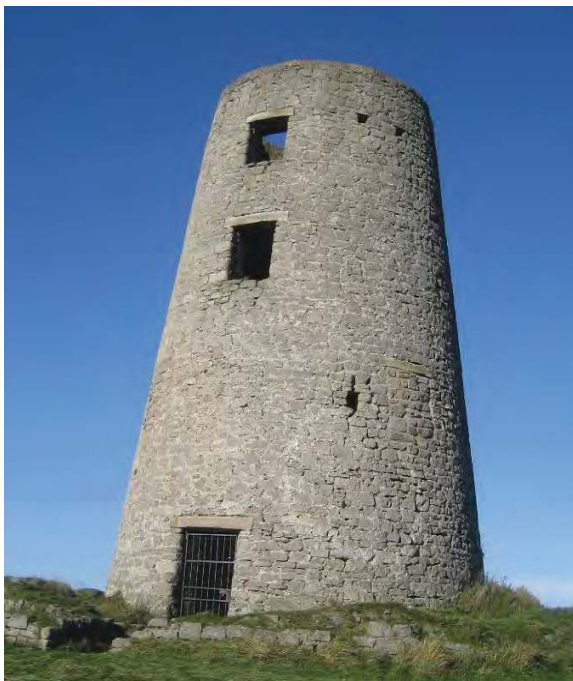
Plate 27: Cleadon Windmill. The walls are of local limestone with Coal Measures sandstone used for door and window lintels.
