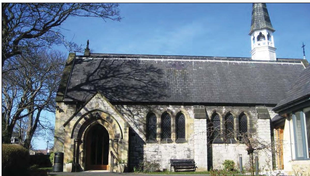
Plate 26: All Saints Church. The walls of the original church are built mainly of local limestone, though sandstones are employed as quoins and for door and window casings, with imported Welsh slate used on the roof.
