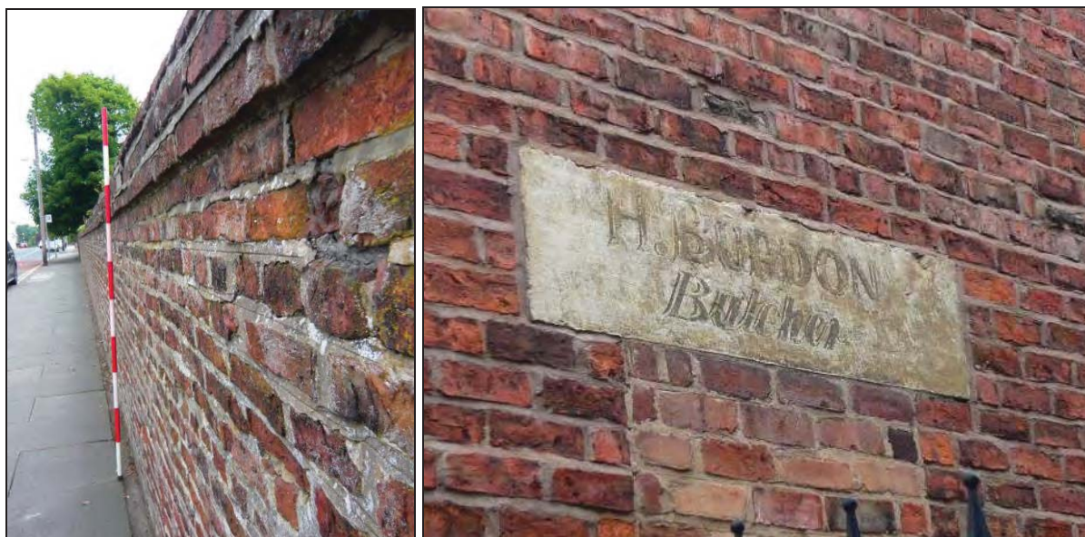
Plates 93 and 94: Local Pelaw Clay bricks used in the 18th Century boundary wall of Cleadon House (left), and the 19th Century gable wall of Grove House (HER 12780) (right); note the different colour and matrix of the bricks used for the later infill in the blocked doorway under 'H. Burdon Butcher.'
