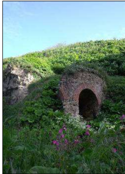
Hawthorn Hive, closer view of late 18 th century twin pot limekiln Still a significant presence but falling into decay..
