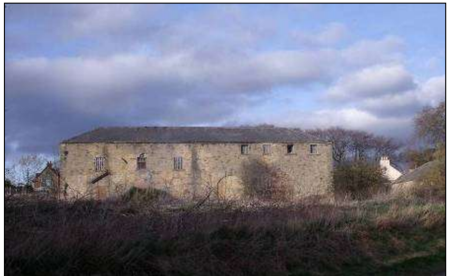
Plate 59. Old Cassop: Former cart shed and byre made of local stone with traditional pantile roof. Now falling into decay. Such vernacular buildings are worthwhile in their own right, but also contribute significantly to historic landscape character. This example overlooks rigg and furrow cultivation, historic hedges and dykes which collectively are the distinctive elements of the Limestone Landscape historic character.
